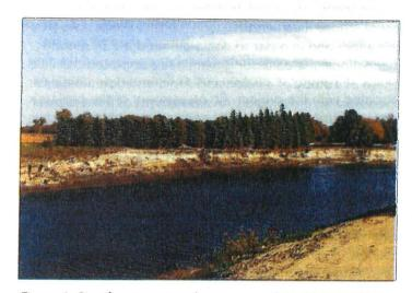
Figure 1: Significant erosion downstream of the Highway 41 bridge at Velva is illustrated by the proximity of the pine trees to the riverbank—before the 2011 flood, about 300 feet of land stood between these trees and the river
