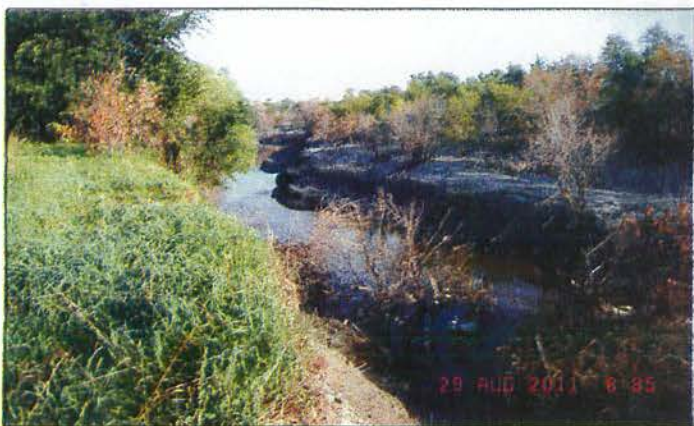
Figure 11: The most severe erosion in 2011 occurred where levees or steep valley slopes constricted the flow of water, such as this point on the Des Lacs River in Burlington
