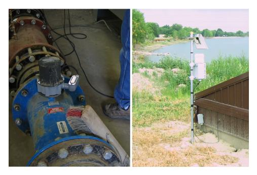
Figure 4. Installation of IDT Telemetry at the Schaper Water Depot owned by Jim Schaper. Exterior view of the telemetry system, with the hand-held calibration system.
