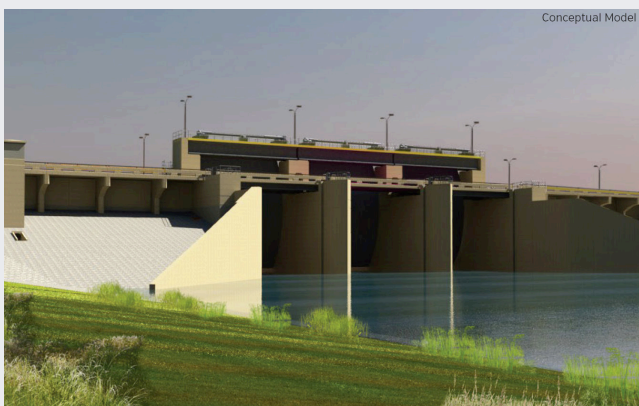
The United States Army Corps of Engineers preliminary design concept model of the FM Area Diversion Project Red River Control Structure.
