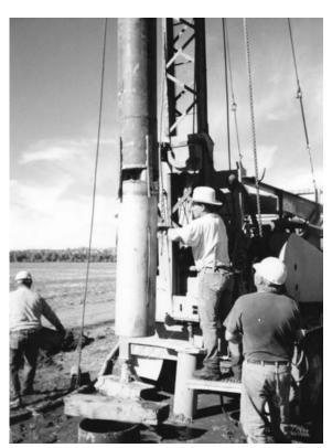
Lako Drilling places cylinders for measuring natural nitrate removal rates in the Elk Valley aquifer, a joint project of the University of ND and the NDSWC.
