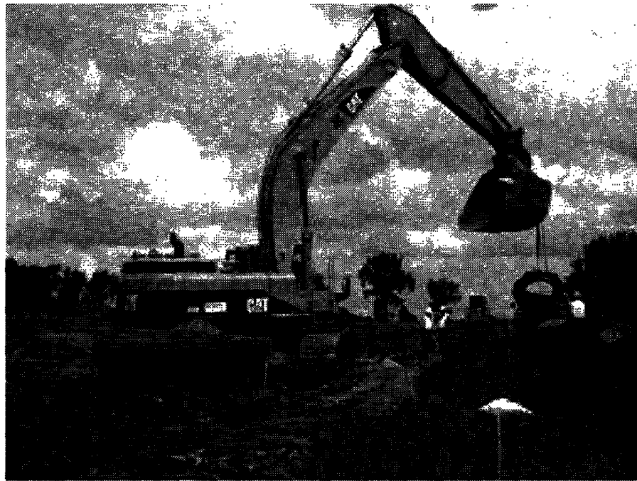
Construction south of Minot on Northwest Area Water Supply project.
