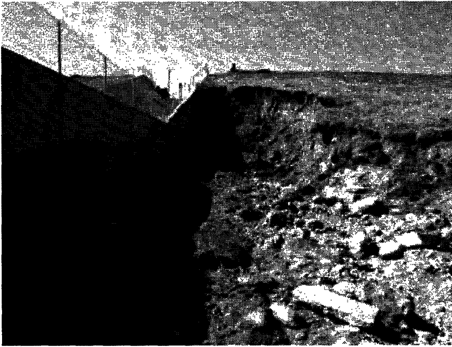
Mount Carmel Dam, showing erosion of the embankment.
