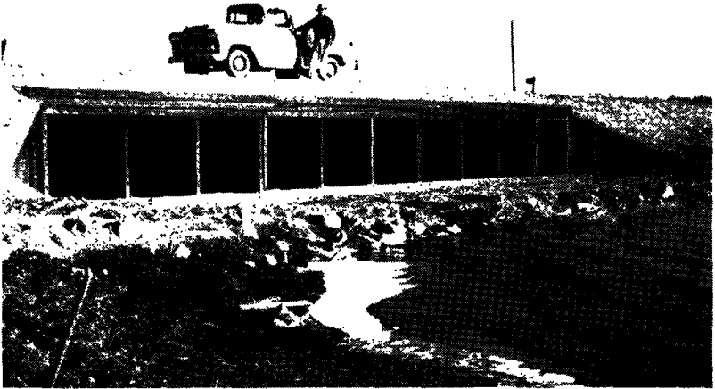
Ziebaugh Pass Culvert Installation
