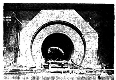
Floodlights enabled the photographer to take this night picture of the upstream portal of tunnel No. 7, recently completed. This tunnel is 22 ft. in diameter and required 10,947 cubic yards of concrete in the  $3\frac{1}{2}$  ft. thick lining.
