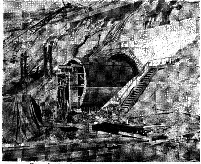
Form for 3<sup>1</sup>/<sub>2</sub> ft. Concrete Lining, Garrison Tunnel
