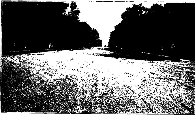
Gravel surfacing in Ransom county, F. A. P. No. 28-C. This section is just outside of Lisbon and part of State Highway No. 9.
