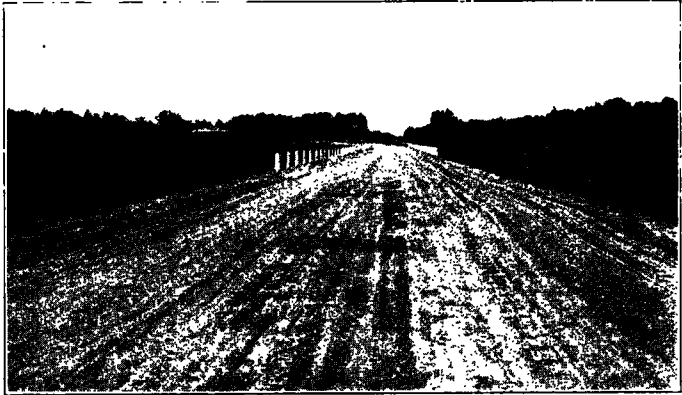
Earth grading in Rolette county on State Highway No. 5, the most northerly of the east and west roads. F. A. P. No. 196. Observe the guard railing on both sides near the turn for protection of the traffic.
